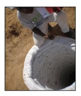
The walls of the pit should be supported, where required, with materials such as sand bags, bamboo poles, corrugated sheeting, concrete culverts and so on.
